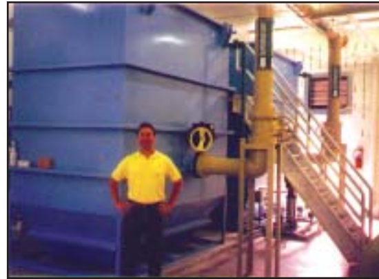
Consultant, Paul Gross, of Buchart-Horn Inc. is standing in front of Smithburg's two (2-disk) AquaDisk filters.
