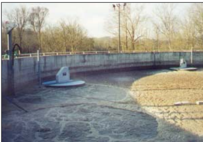
One of the two AquaSBR basins during the React Phase of treatment.
