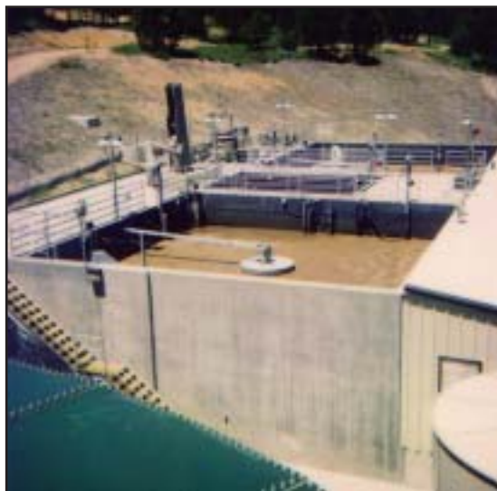
Hume Lake's two SBR basins are located side-by-side with the exception of an aerobic digester basin and blower room inbetween them. Each SBR basin is 36 x 36 x 15.1 feet.
